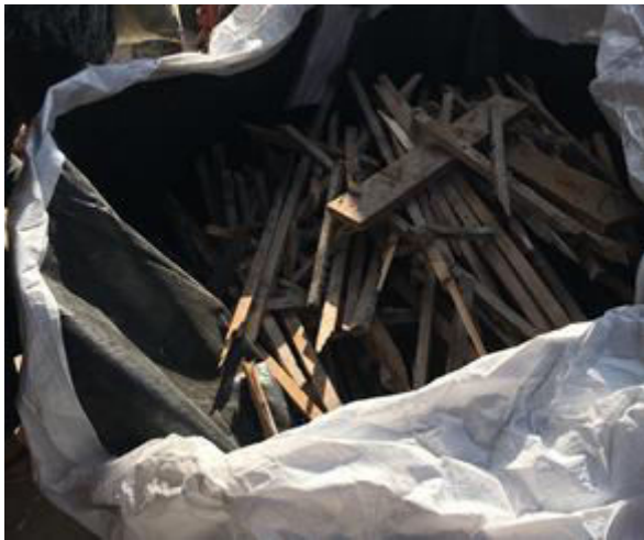
Figure 3. Wooden slats removed from an historical bole house in Visby (the same property as in Fig. 2).
